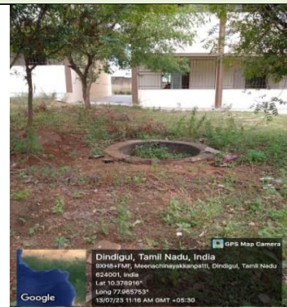
Rain Water Harvesting Pit - 9
