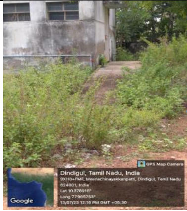
Rain Water Harvesting Pit - 10
