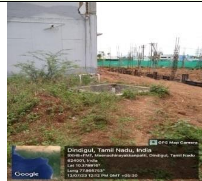
Rain Water Harvesting Pit - 6
